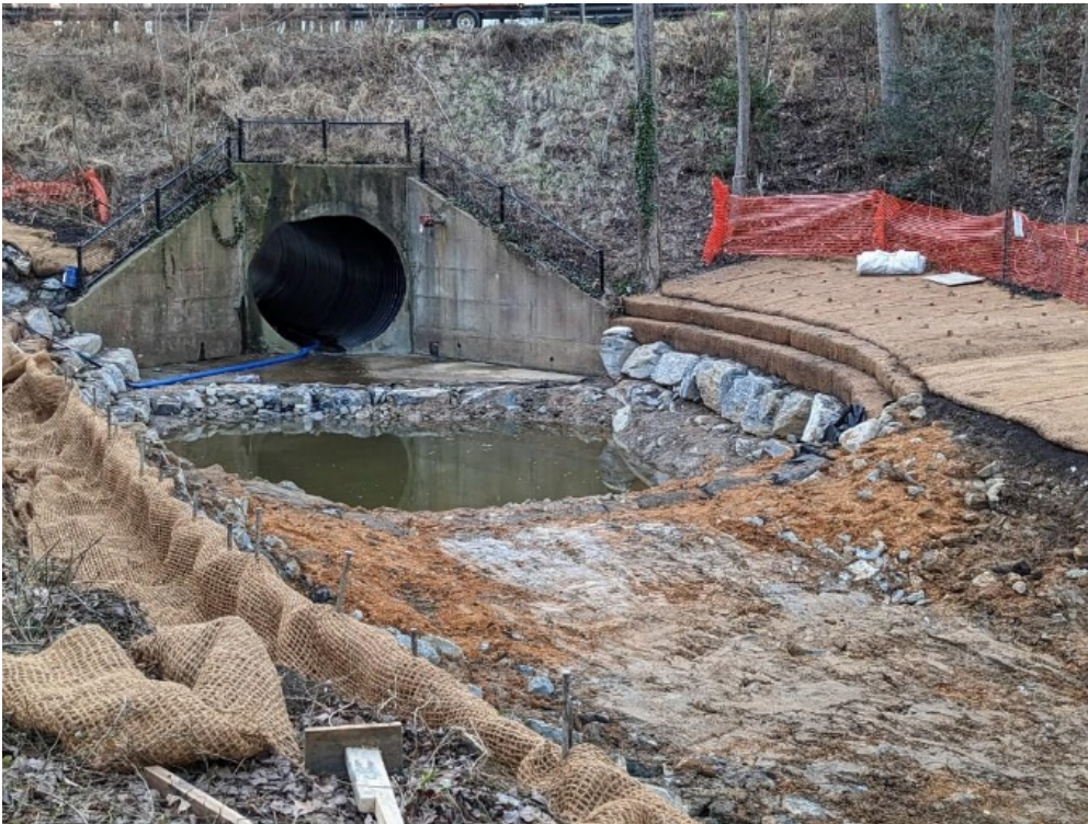
Plunge pool construction at the Fenway Road culvert
